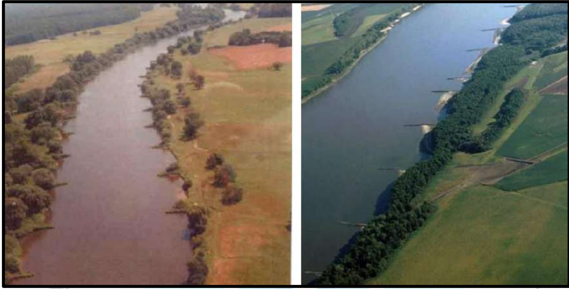
Figure 1. Bidirectional and unidirectional spur applications a) Odra River (Poland) b) Mississippi river (USA) (Özyaman, 2016)
